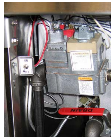
Figure 5: Tuck the wires behind the switch.
